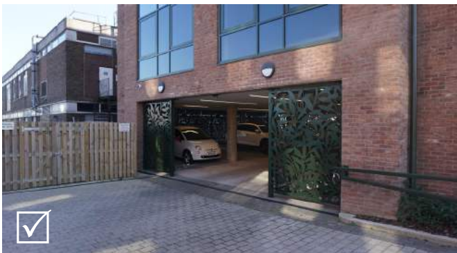
Entrance to parking area under apartment block is made discrete by attractive metalwork panels
