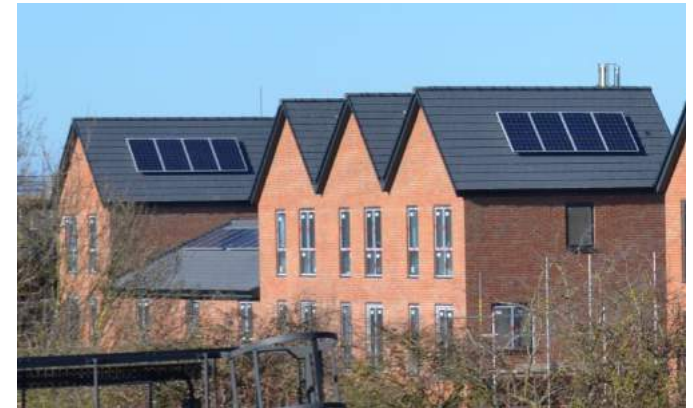
Solar panels at Brooks Mews, Aylesbury
