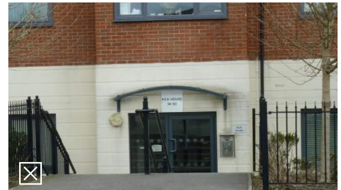
Building entrances should be at street level, or slightly elevated but not below street level
