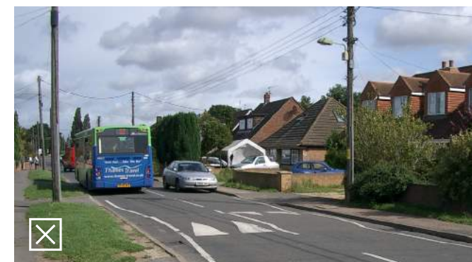
Speed bumps as a traffic calming measure for new roads should be avoided.
