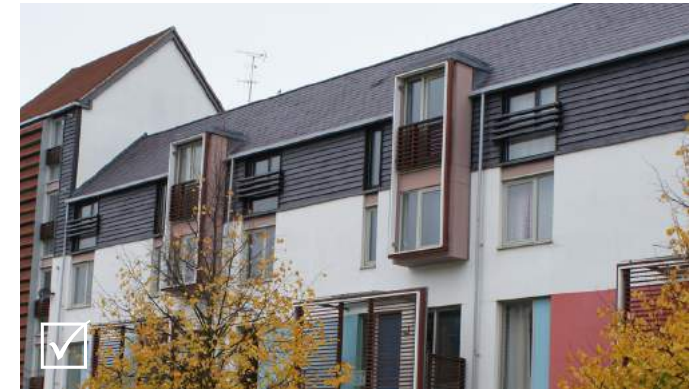
Dormers can be used in new development to reflect local vernacular in a modern way. Avoid dormers that are out of proportion with the facade
