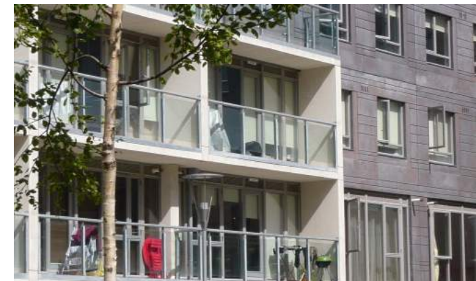
Recessed balconies provide additional privacy to the rooms that open onto them
