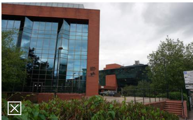
Office building is set back from the street and the entrance is not obvious
