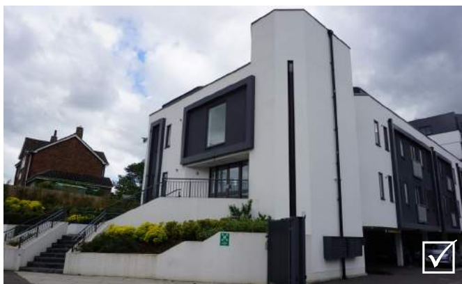
Conversion of Ringwood House, Aylesbury, from office to residential use. The conversion remodels the entrance and gives the building a contemporary feel
