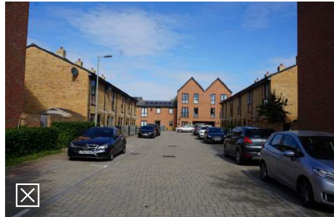
A residential street with little planting results in a hard environment, dominated by cars
