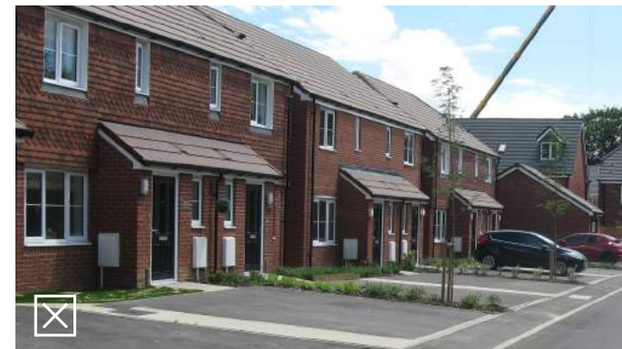
Meter boxes are prominent on building frontages
