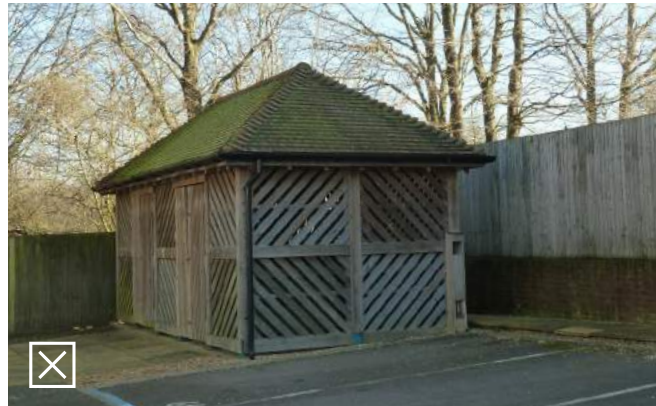
Bin stores is located within parking spaces and appears to be an afterthought
