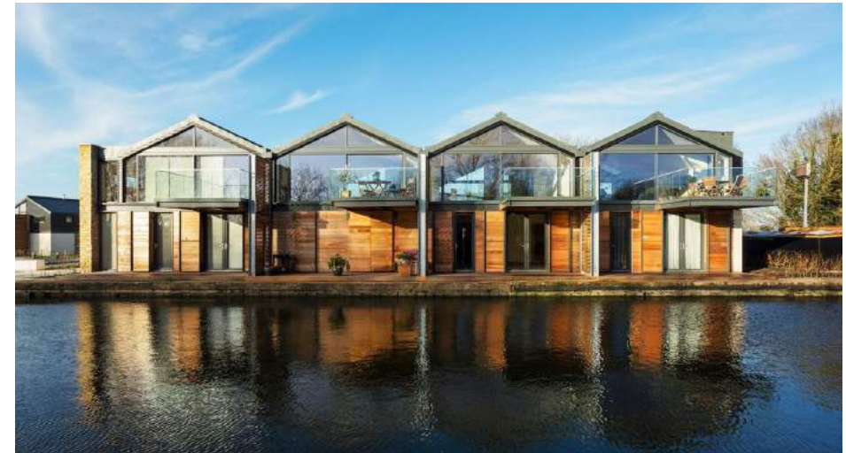
New residential dwellings at Marsworth Yard front onto the canal and have been designed with a contemporary wharfside architectural style
