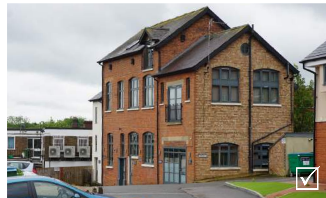
Former warehouse building in Buckingham converted to residential use
