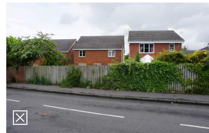
Properties expose their rear boundaries to the street providing no animation or overlooking of the streetspace and contrary to secured by design principles
