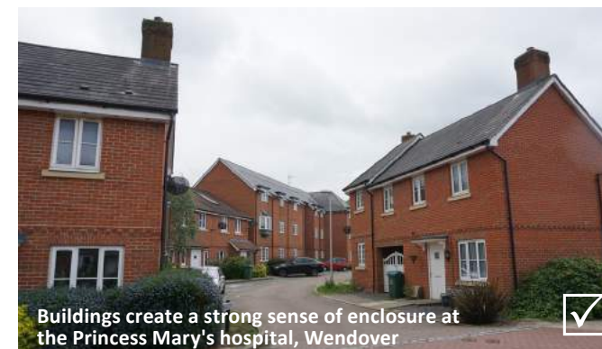
Buildings define the back of footway at the former Princess Mary's hospital, Wendover
