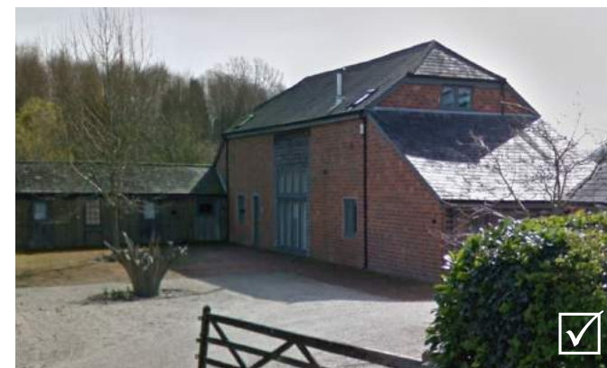
Successful retention of existing openings
