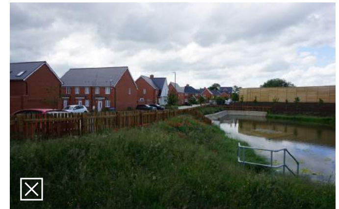
Attenuation pond is poorly integrated into the residential development so that it has limited visual amenity value
