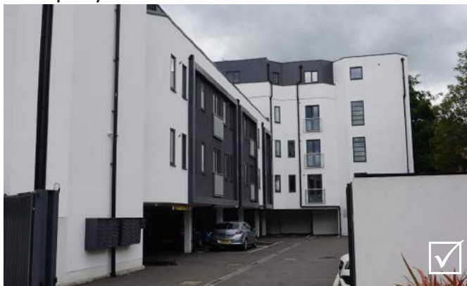
Conversion of Ringwood House, Aylesbury, from office to residential use - car parking is within an undercroft where it is hidden from the street
