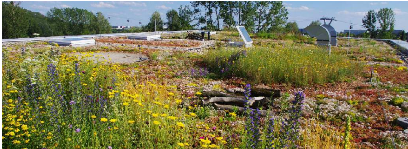
A bio-diverse (brown) extensive roof
