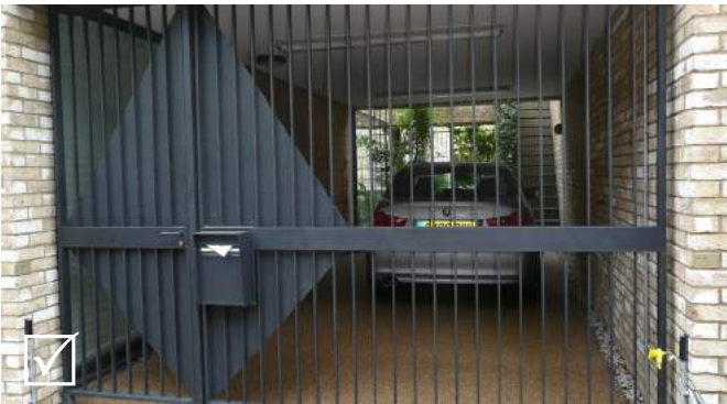
The use of gates rather than garage doors can be beneficial in ensuring the space is used for parking cars and not storage
