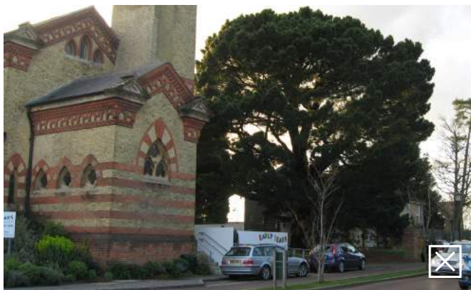
Entrance to nursery is not designed to be respectful of the historic chapel
